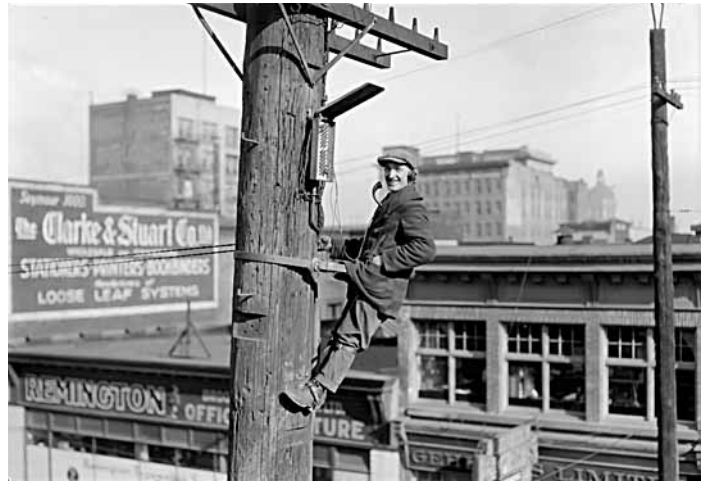
BC Tel Lineman 1927
