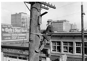
BC Tel Lineman 1927
